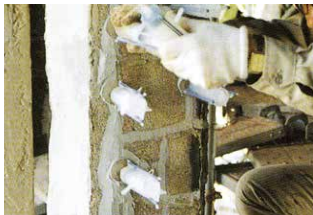
柱ひび割れ補修
