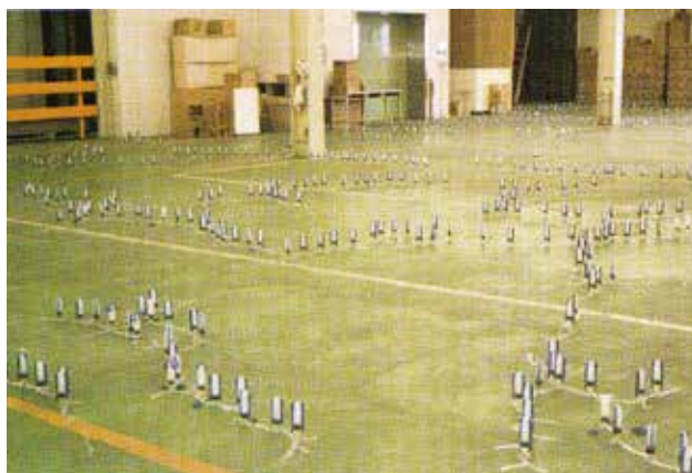
床ひび割れ補修
